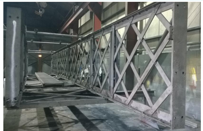
The lattice section of the footbridge has been removed and is now at our workshop in Cardiff
